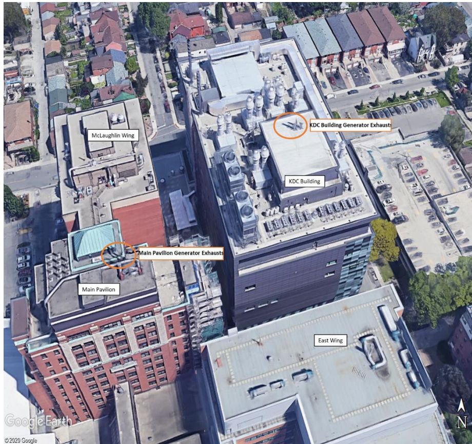
Figure 2: Generator Exhaust Locations
